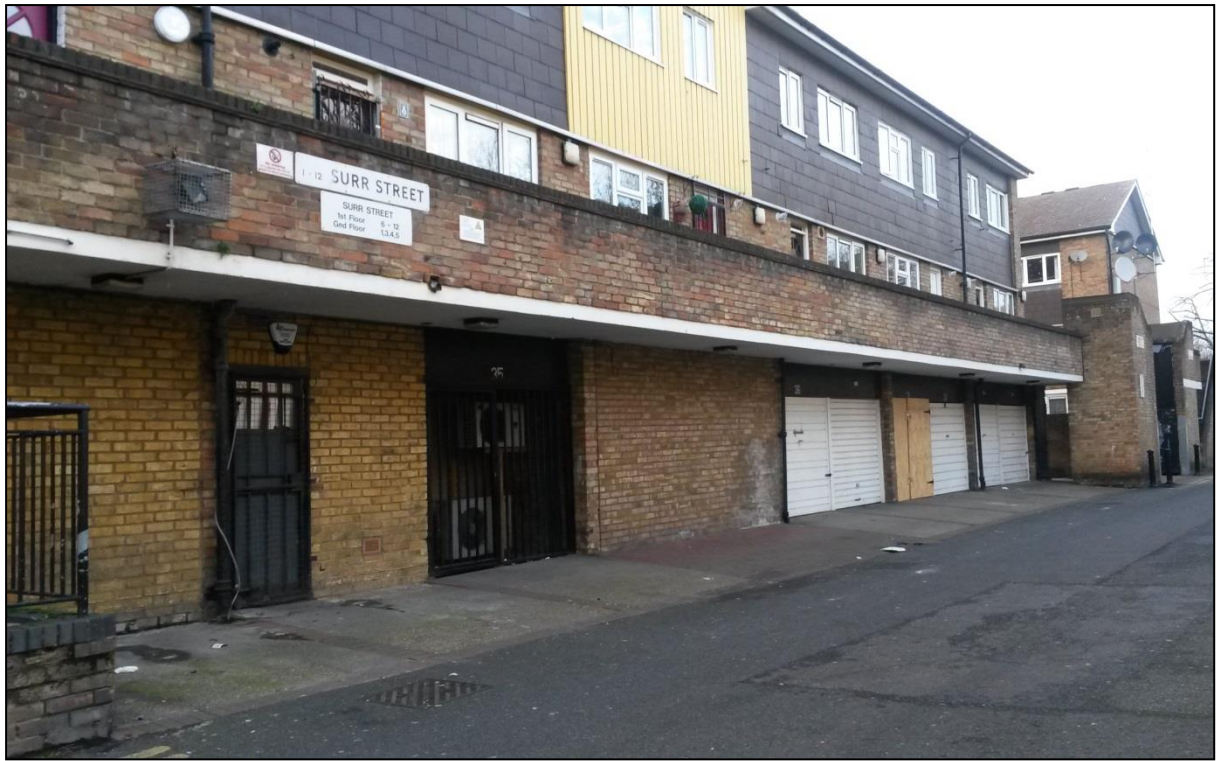
Fig. 4: Garages beneath 1-12 Surr Street ("Site 2a")
